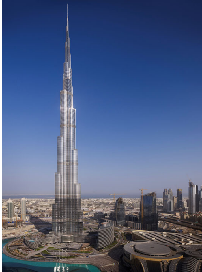
Figure 1.4 The Burj Khalifa, the current tallest structure in the world.
