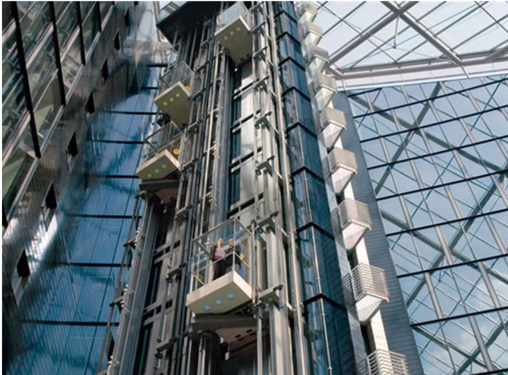
Figure 13.4 A multideck twin elevator system.
