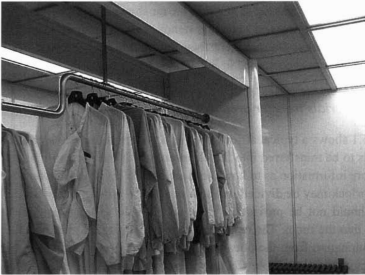
Figure 5.7 Cleanroom clothing under a vertical unidirectional airflow
