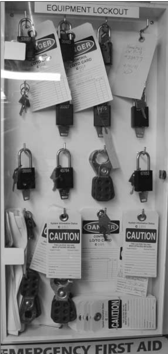
FIGURE A.1 Lock-out/tag-out center.
