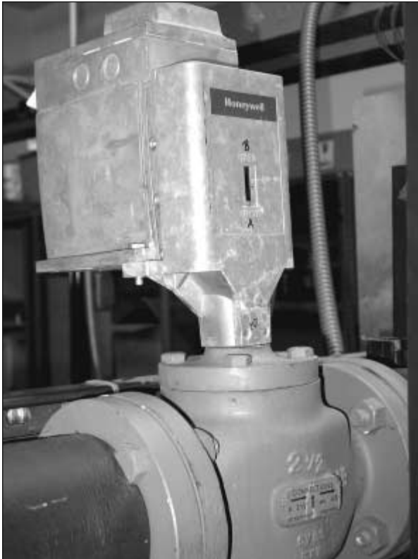
FIGURE 5.42 Electronic valve actuator and valve housing.
