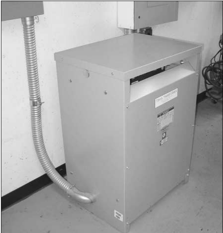
FIGURE 4.16 750 kVA Transformer.
