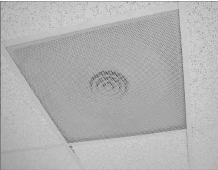
FIGURE 16.9 Zone air diffuser.
