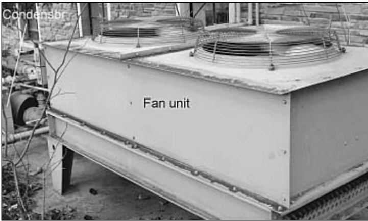
FIGURE 9.4 Dry cooler.
