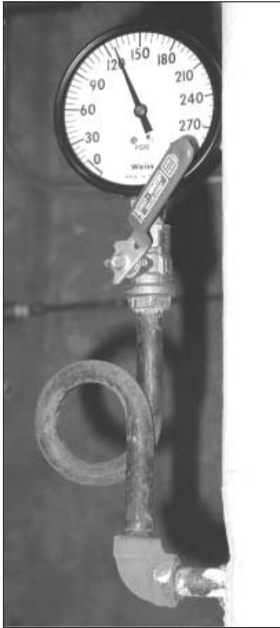
FIGURE 12.16 Steam pressure gauge with protective loop.
