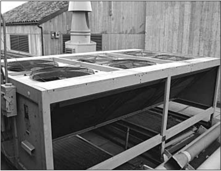
FIGURE 9.2 Typical air-cooled condenser.
