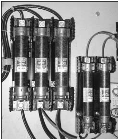
FIGURE 4.18 Fuse bank.
