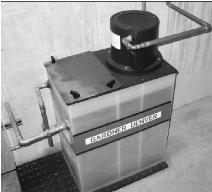
FIGURE 2.16 Water/oil separator.
