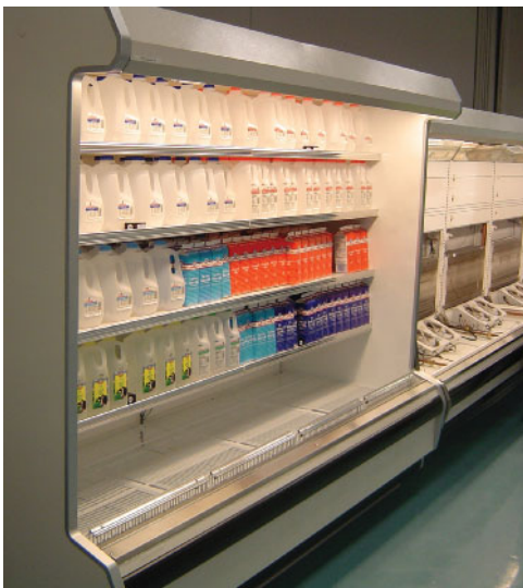
Figure 10-1 Open front refrigerated case at the Hussmann Training Center. Courtesy of Hussmann Training Center.
