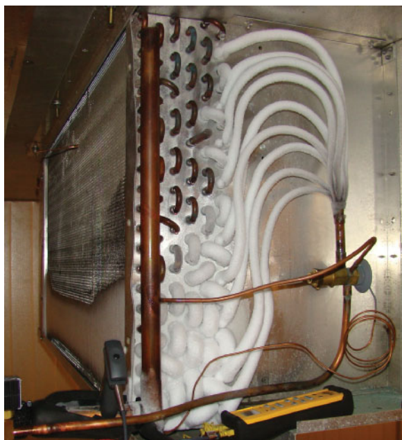
Figure 11-25 Evaporator with refrigeration problems will have uneven frost buildup (left) and a freezer evaporator that is overdue for its defrost has even frost buildup (right). Photos by Dick Wirz.
