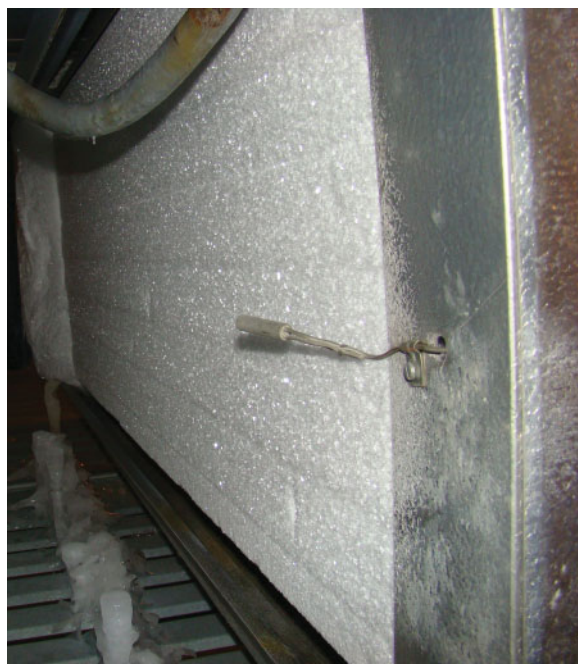
Figure 11-25 Evaporator with refrigeration problems will have uneven frost buildup (left) and a freezer evaporator that is overdue for its defrost has even frost buildup (right). Photos by Dick Wirz.
