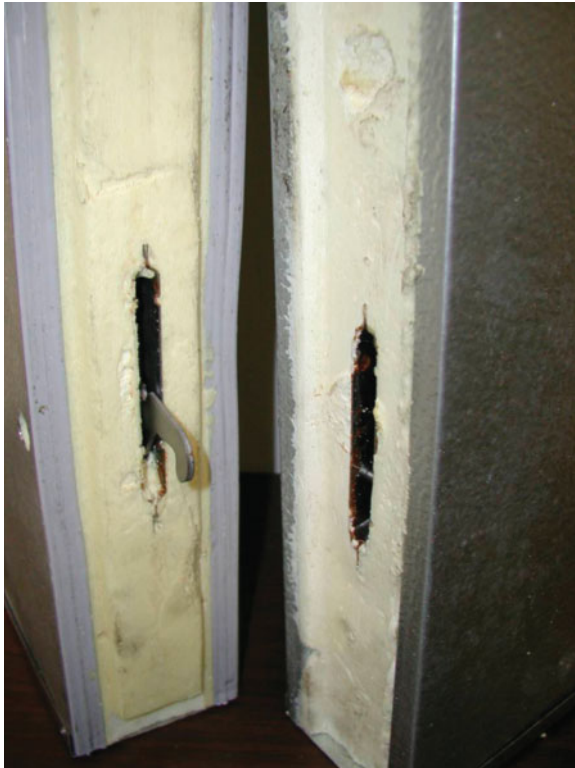
Figure 11-1 Walk-in panel locks foamed in place (left) and locks in wood framing (right). Courtesy of Jerry Meyer, Hussmann Learning Solutions.
