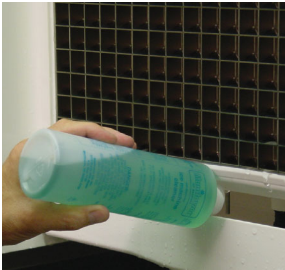
Figure 12–9 Use cleaner and a brush to clean ice machine evaporators. Courtesy of Manitowoc Ice, Inc.
