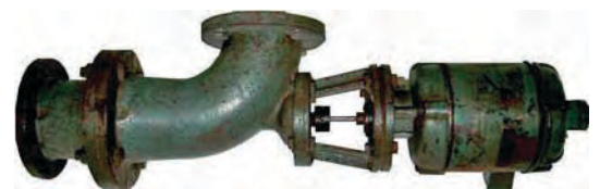
First heating circulating pump, the “elbow pump”, model year 1929, HP type DN 67/0.25 kW
